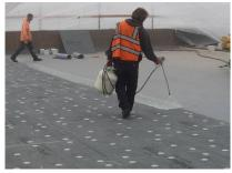
➤ The project replaced the 1.2-acre roof (which happens to be larger than most residential lots in either Juneau or Sitka) with a 90-mil EPDM membrane, drainage, and overflow structures. The construction included abatement of nearly 5.8 tons of asbestos and has not had a change order.
