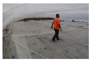
The existing 53,000 square foot built-up roof was approaching 50 years old and showing significant signs of deterioration. Pooling water could be seen on roof sections from satellite photography and leaks were common to navigate around when servicing aircraft.
